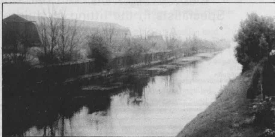
The old course of the Nene, looking towards March, with the piles of the old wharf against the far bank. The small building in the centre is the goods office of Benwick's abandoned station.
