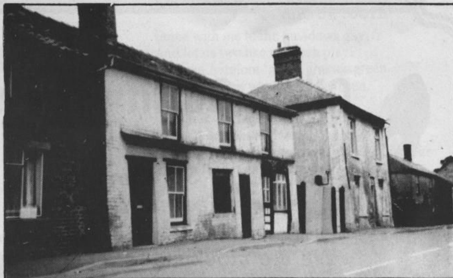
Buildings in the High Street. Note how doors and windows have been rehung vertically to counteract the tilting of the house.
